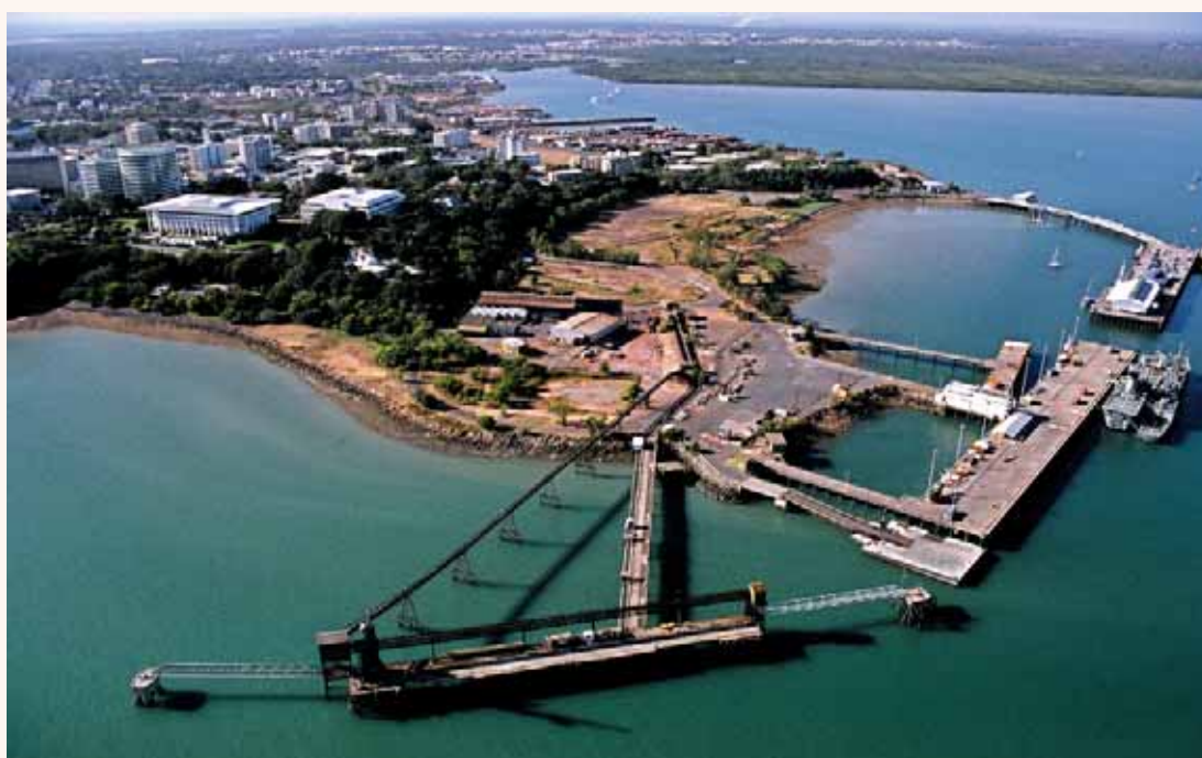
Aerial view of the Darwin City Waterfront Project, Northern Territory
